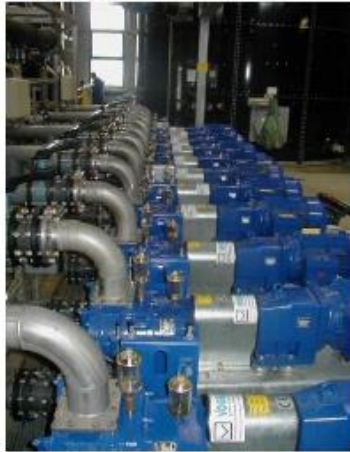
Beverage processing line 饮料加工线
