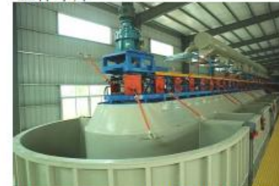
Electroplating production line 电镀生产线
